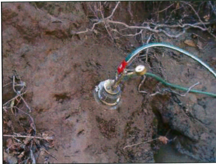
Typical installation of jet testing equipment in stream bank
