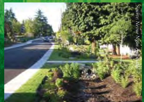
Figure 5-5: When a street is completely reconstructed, such as the Street Edge Alternatives (SEA) Streets in Seattle, Washington, the project uses a full-integration approach.
