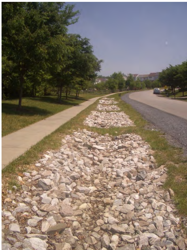
Rural Highway Infiltration Trench
