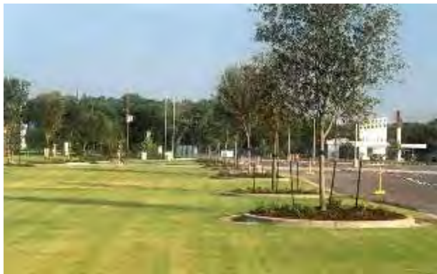
Figure 53. Reinforced turf used as overflow parking area. Source: Cahill Associates
