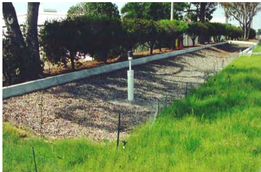
Figure 78. Infiltration Trench. Source: RBF Consulting
