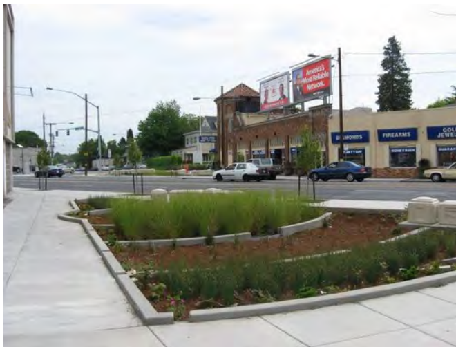
Figure 2. This bioretention area takes runoff from the street through a trench drain in the sidewalk as well as runoff from the sidewalk through curb cuts (Source: Abby Hall, US EPA).
