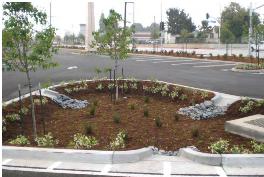
Figure 29. Newly Planted Bioretention Cell in El Monte, CA.
