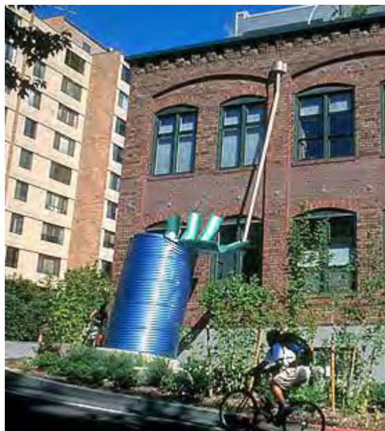
In this functional sculpture, a cistern captures roof runoff and drains it slowly to a landscaped area. Photo courtesy of the City of Seattle.
