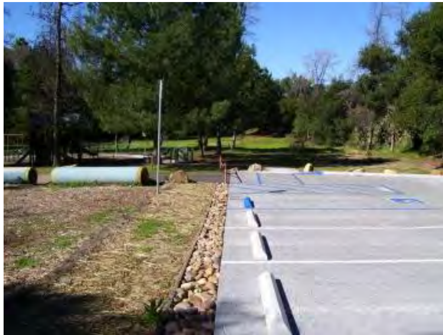
Figure 55. Pervious concrete parking lot with river stone edge treatment at Flinn Springs County Park, El Cajon, CA.
