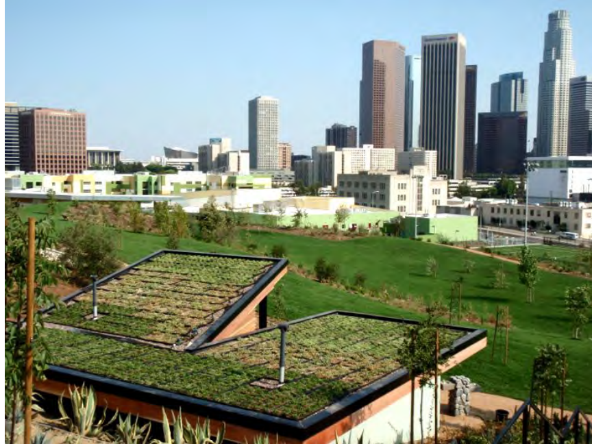
Figure 69. Vista Hermosa Park Ranger Station, Los Angeles. Source: Greenroofs.com
