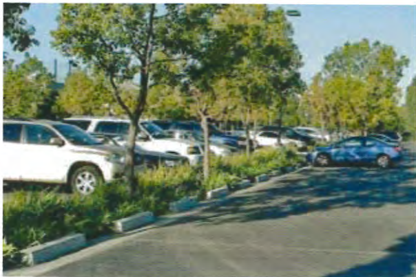
Vegetated swale in a parking lot
