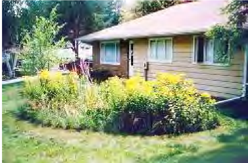
Figure 19. Roof leader draining to bioretention cell. Source: Wild Ones Natural Landscapers, Ltd., Applewood, MI.
