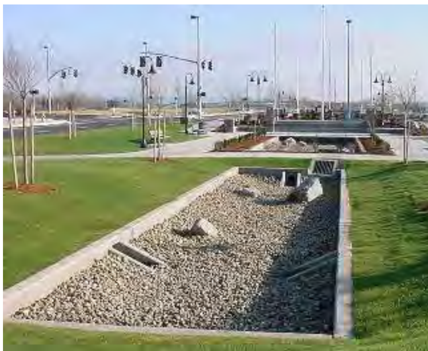
Figure 82. Surface media filter. Source: Portland BES
