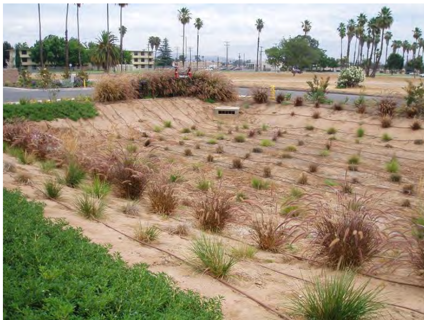
Figure 77. Infiltration Basin. Source: March Joint Powers Authority
