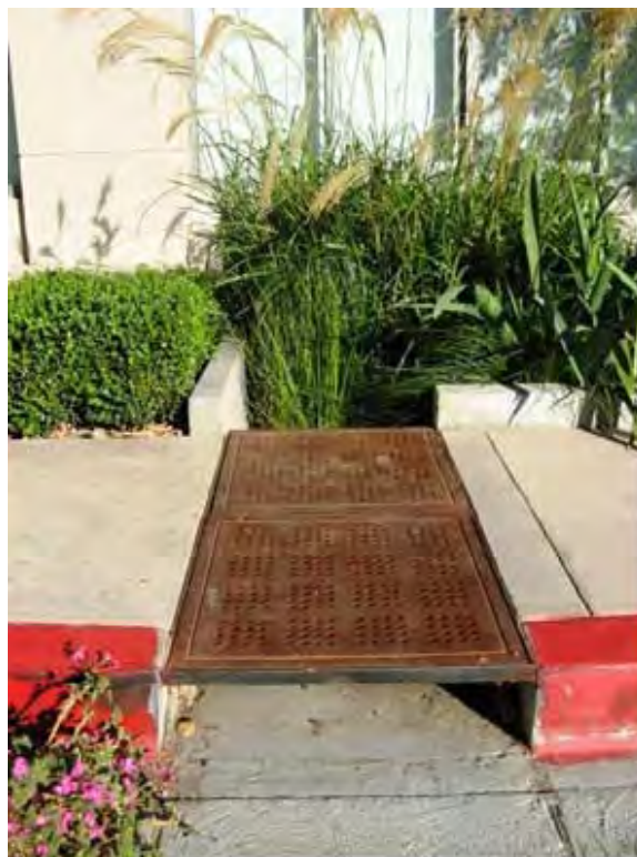
Figure 25. Curb cut directing water from the street into a bioswale. Source: Haan-Fawn Chau
