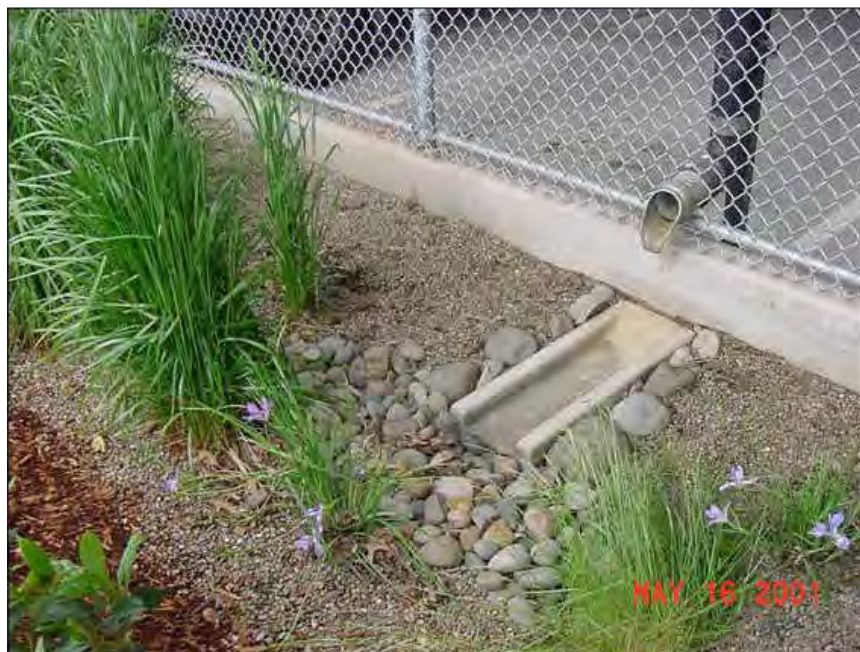
Figure 72. Downspout disconnection into vegetated area. Source: Prince George's County, MD Department of Environmental Resources
