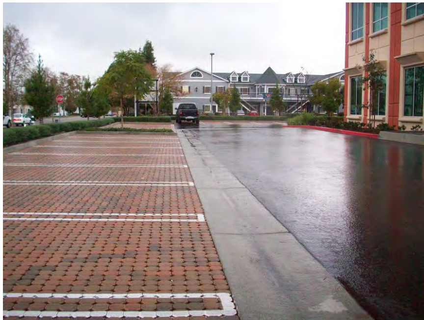
Figure 33. Pervious Paver Parking Stalls, Redlands, CA. Source: Jeff Endicott
