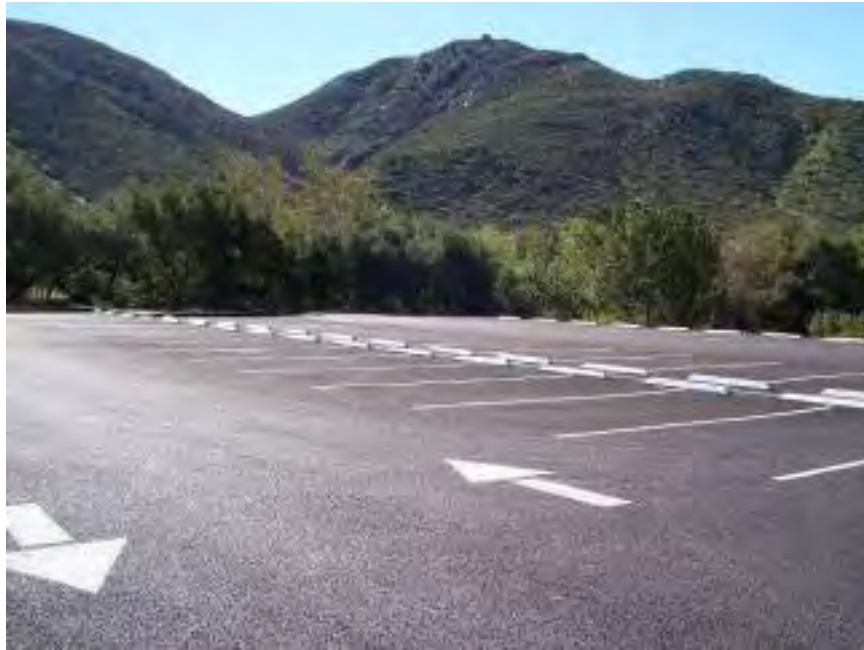
Figure 40. Pervious asphalt parking lot at Flinn Springs County Park in El Cajon, CA. Source: Cahill Associates
