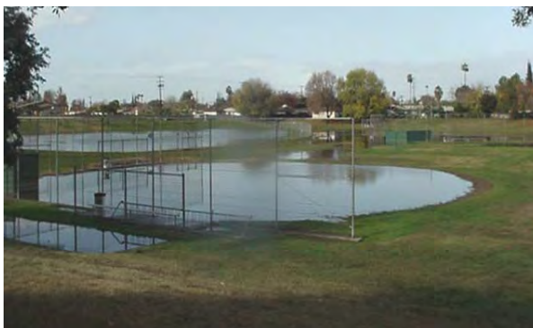
Infiltration Basin in a Fresno, CA Park, Before and After a Rain Event
