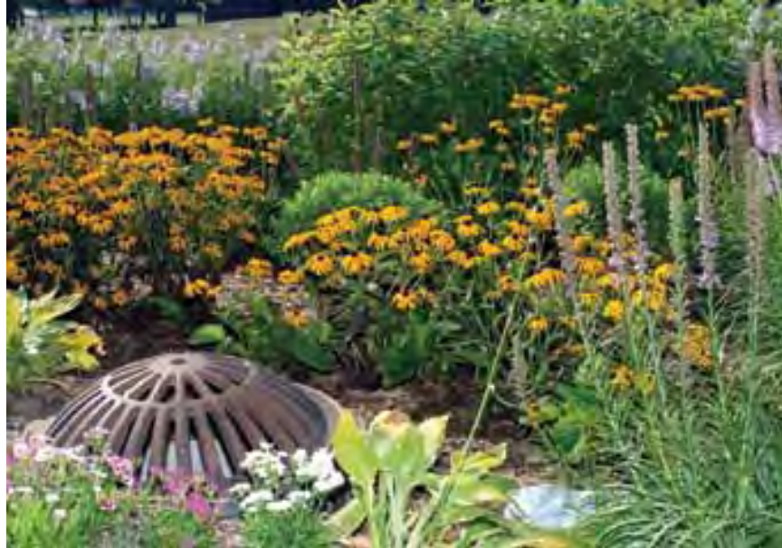
Figure 26. Positive Overflow Device: Domed Riser. Source: Macomb County Michigan Public Works Office
