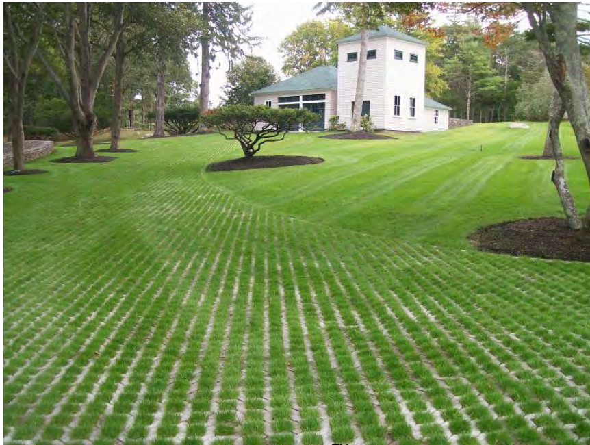
Figure 45. Turfstone™ Driveway. Source: Nicolock
