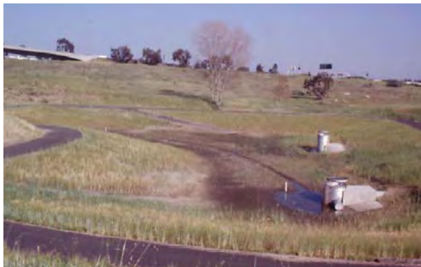
Figure 80. Dry pond. Source: RBF Consulting
