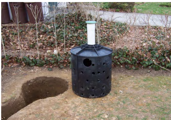
Drywell installation
