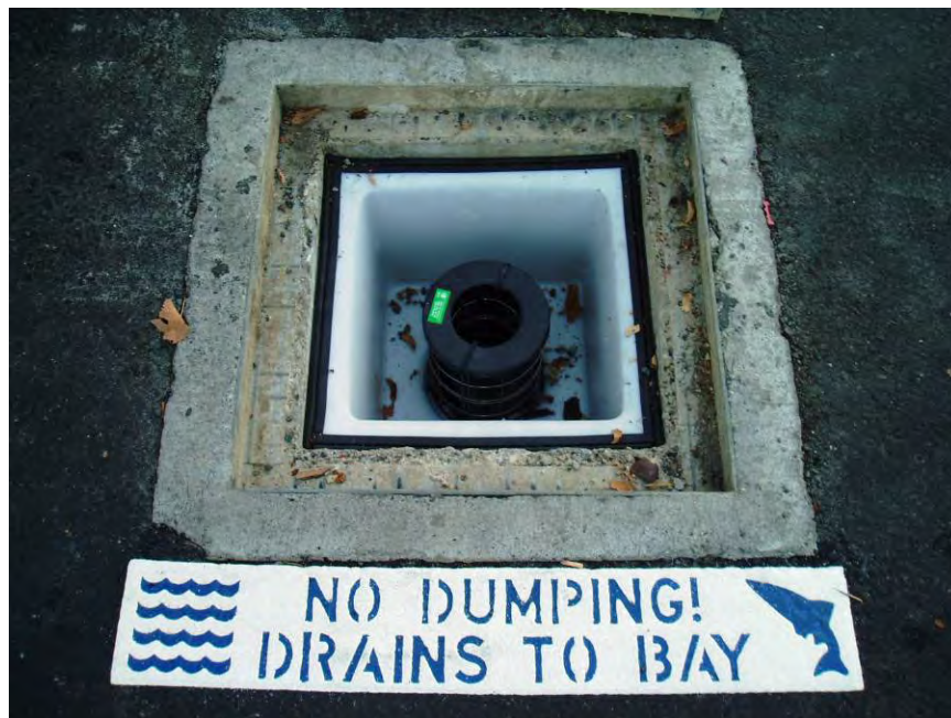
Figure 83. Catch basin insert. Source: REM Inc.
