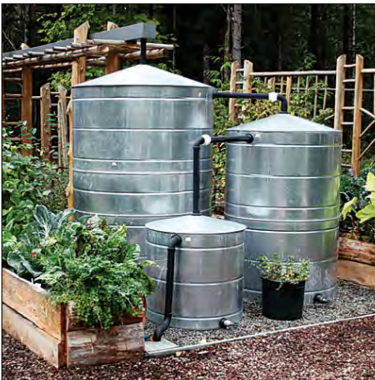
Figure 61. Cisterns used for irrigation. Source: Sunset Publishing Corporation
