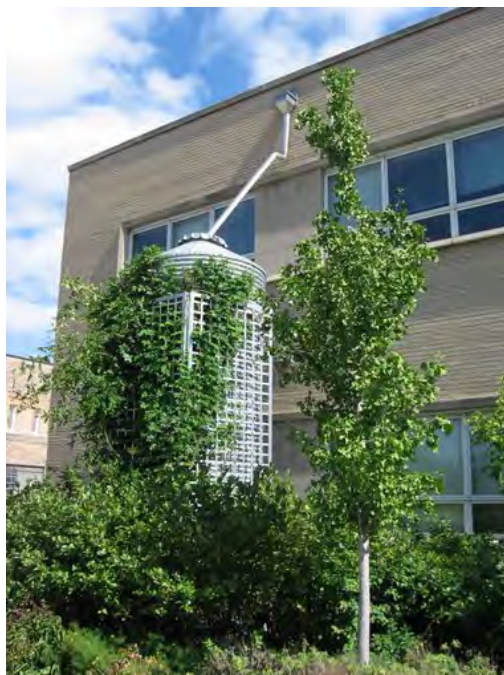
Figure 5. Rain water cistern.
