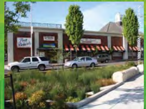
Figure 5-4: The five rain garden projects located along NE Sandy Boulevard in Portland are located where the site constraints were minimal
