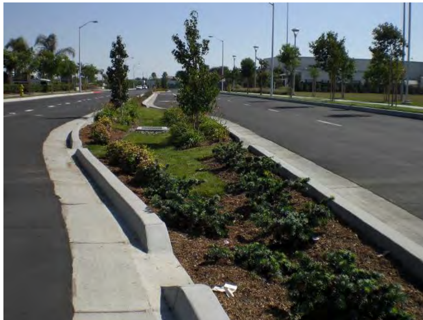
Figure 24. Bioretention cell for street/yard drainage, Downey, CA.
