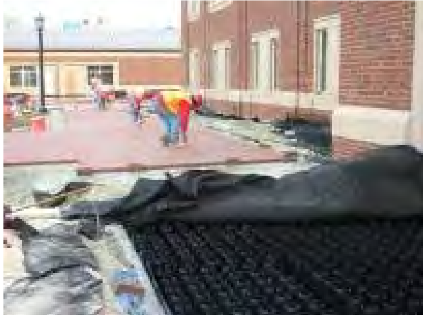
Figure 66. Rainstore™ unit beneath brick pavers on a vegetated rooftop plaza. Source: Cahill Associates
