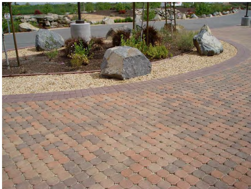
Figure 34. Pervious Paver Driveway, Chino, CA.
