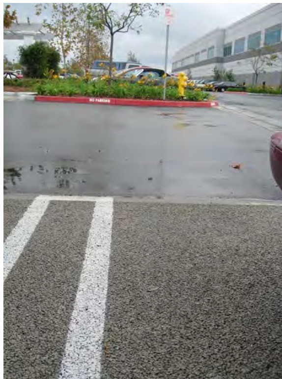
Figure 43. Pervious concrete parking areas, Haas Automation, Inc., Oxnard, CA. Source: Lorraine Rubin
