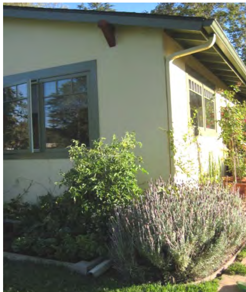
Diverted Roof Runoff City of Santa Barbara
