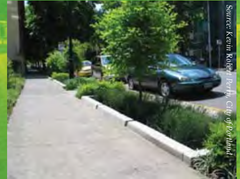
Figure 5-3: Portland's SW 12th Avenue Green Street project utilizes a strategic approach in placing smaller stormwater facilities intermittently along the streetscape
