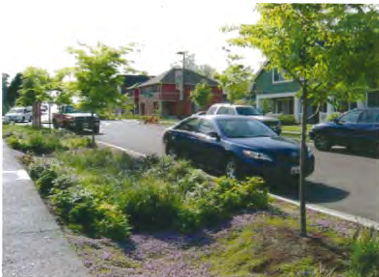
Drainage swale as part of Seattle’s SEA (Street Edge Alternatives) Project / CREDIT: EPA/ Abby Hall
