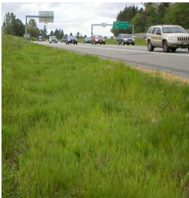
Vegetated filter strip captures runoff from freeway
